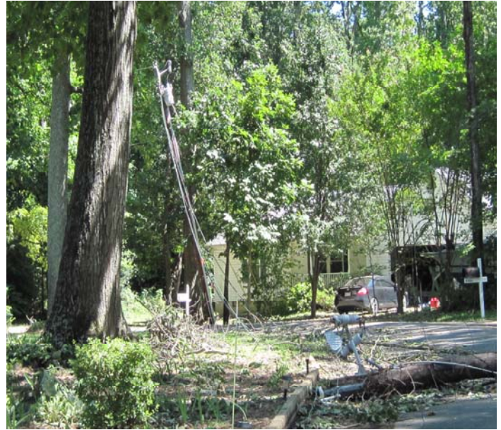
Shocking? Perhaps - The danger, in this example, is the downed electric power line entangled in trees. Until declared "dead" by SMECO, downed lines such as this must be considered "life threatening" and not touched by the layman.
