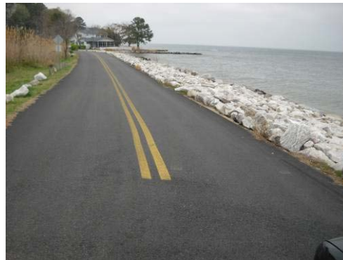
Causeway asphalt and revetment
