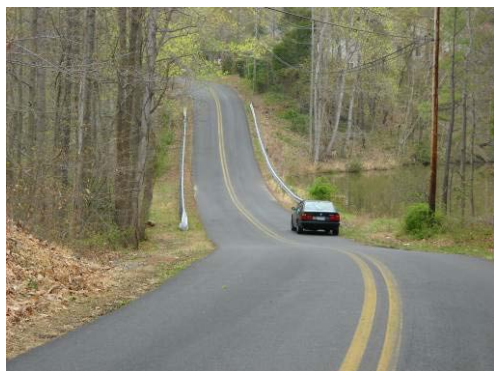
Roadway at causeway with guard rail
