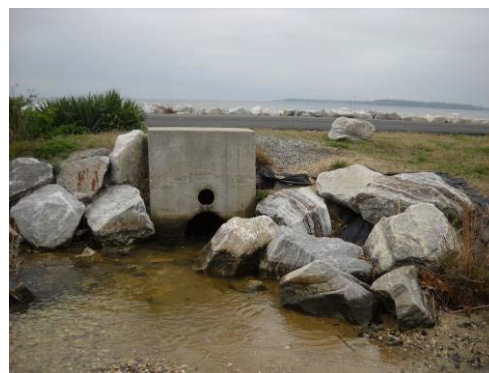
Replaced tidal pond culvert & headwall at causeway
