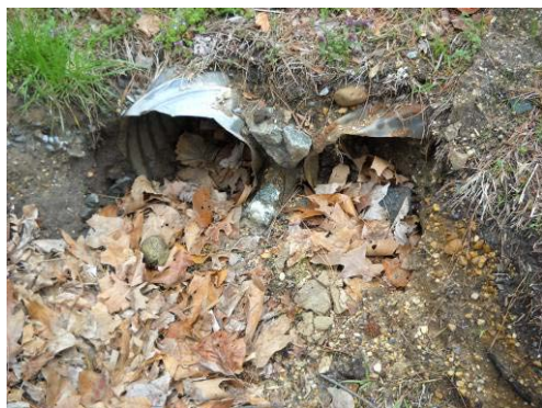
Damaged culvert
