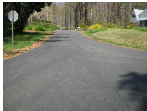
Typical roadway surface
